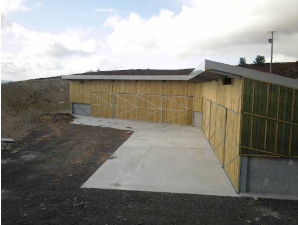
Fig.6- Wood chip building as constructed showing concrete apron and sliding doors
