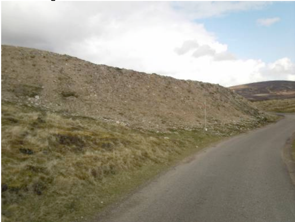
Fig.7- Photograph showing earthworks adjacent to Dorback Road
